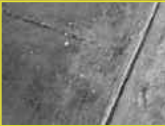
• Concrete Floor Joints
