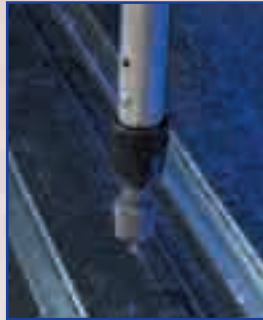
Drill deck holes
